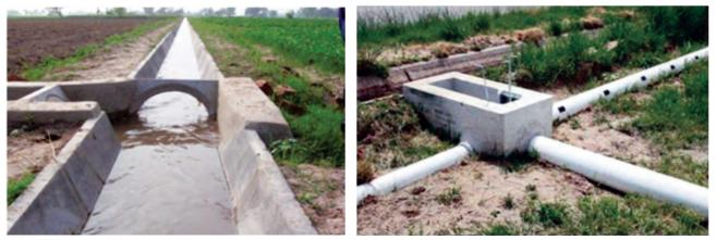
Surface lined (left) and piped water (right) conveyance systems save water and energy and improve the crop yields.
